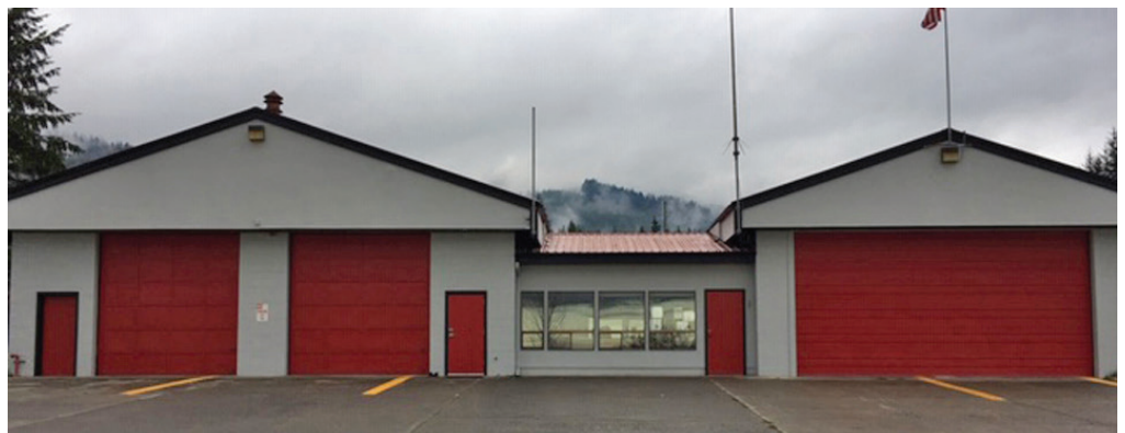
The next major project for the fire district is replacing the primary fire stations in Gales Addition (Station 21), pictured above, and Dry Creek (Station 22), pictured below.
